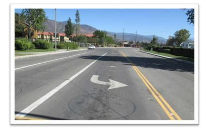
College Avenue is one of the original 47 locations that was approved to Matich Corp for a grind and overlay of asphalt. The City came in after with a Stripping contractor and a Signal loops contractor to complete the improvements seen here.
